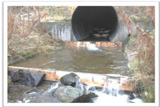
*The Toddle Burn easement was installed in 2016 in a bridge culvert at the bottom of the burn. It resulted in a significant increase in juvenile Trout production upstream of the culvert*
